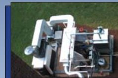
Combined heat and power systems providing electric or shaft power and thermal heat recovery
